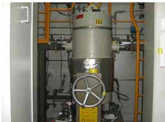
Figure 1: Ion exchange filter of the heavy water system with a heating jacket for the drying of the ion exchange resins.
