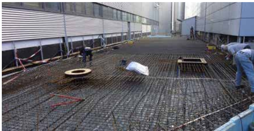
Figure 3: Construction works for the connection between the reactor building and the neutron guide hall east.
