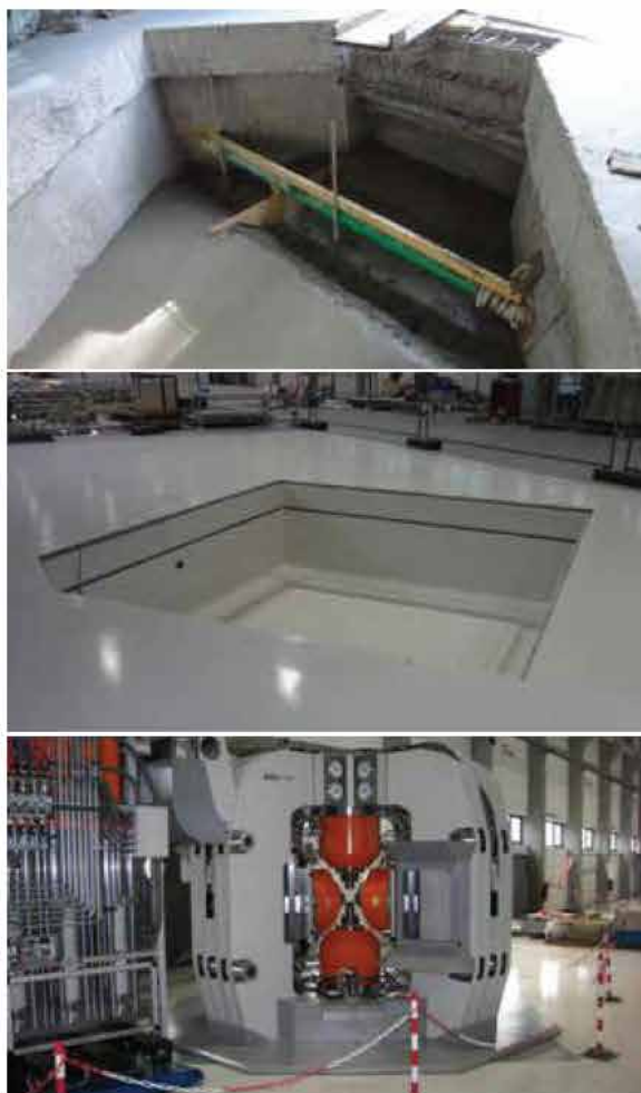
Figure 8: Floor deepening in the neutron guide hall east for the instrument SAPHiR; top: during structural work, middle: finished, bottom: with instrument installed.
