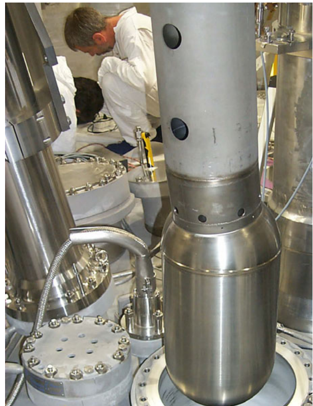
Figure 2: The moderator of the hot source in the reactor pool of the FRM II during installation.
