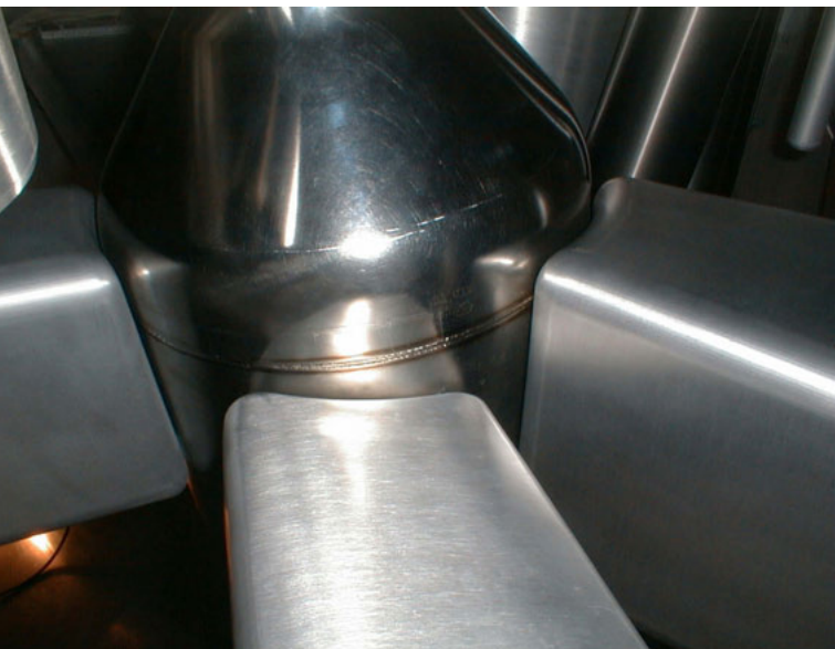
Figure 1: The cold source vessel surrounded by the beam tubes SR 1, 2, 4. View into the moderator tank of the FRM II before operation.
